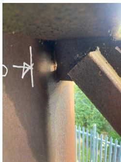
Rack 82, evidence of porosity and lack of side wall fusion.
