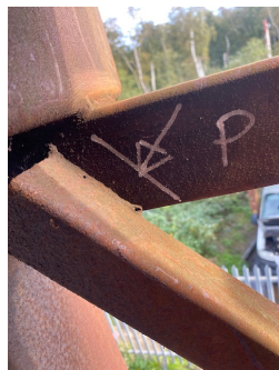
Rack 82, evidence of porosity and lack of side wall fusion.
