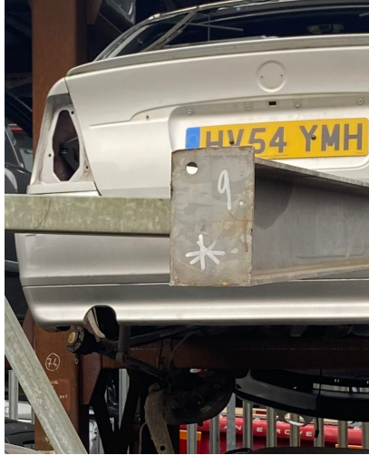
Van/Ebay area, defective racking identification *9 (ie rack number 9 of 10 rejected).
