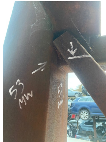
Typical marking/identification of missing welds, ie racks 55 and 53.
