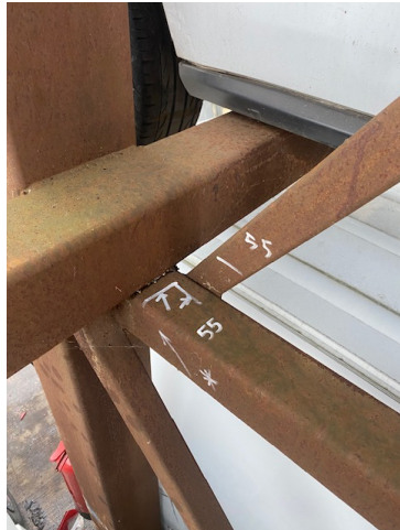
Typical marking/identification of missing welds, ie racks 55 and 53.
